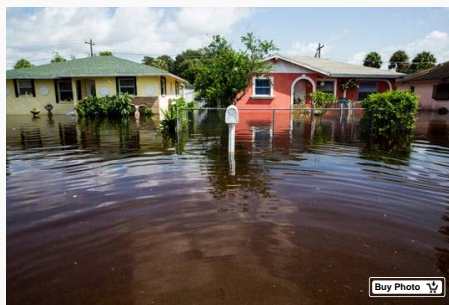
Water floods Pawley Avenue in Bonita Springs on Tuesday, August 29, 2017. The water rose to a few feet in certain places along the street, forcing many families to leave their homes. (Photo: Nicole Rauchslein/ Naples Daily News)
